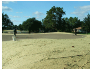
Before hosting qualifying for the PGA Tour's Western Open, the Village Links of Glen Ellyn (Ill.) rebuilt its greens in 2003 to meet USGA recommendations. The USGA recommends that laboratories perform tests on root-zone mixes before seeding begins on a golf course construction project. Photos by Sam Ferro
